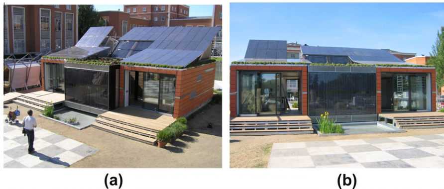
Fig. 1. (a) Birds eye view and (b) south frontage of the solar house.
