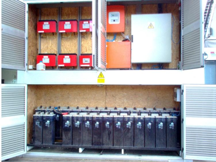
Figure 2.6: Picture of the inverter’s room and battery bank of “MagicBox”, where: red boxes are the five **PV** inverters in use plus one of backup and the upper orange box is the battery inverter.
