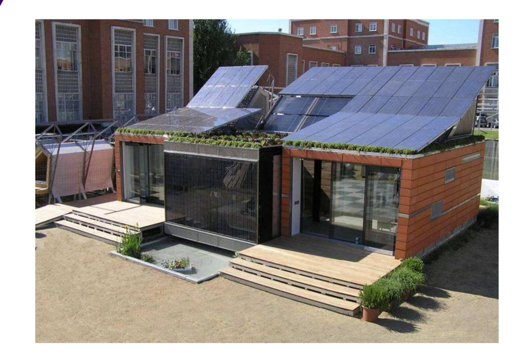
The GeDELOS-PV system is an example of added value for PV electricity arising from the combination of modern hybrid PV technology with a lead-acid battery storage system and Demand Side Management (DSM) strategies in the residential sector. The main objective of this system is to satisfy the user demand by optimizing the use of PV electricity. In order to achieve this objective we have followed two strategies:
